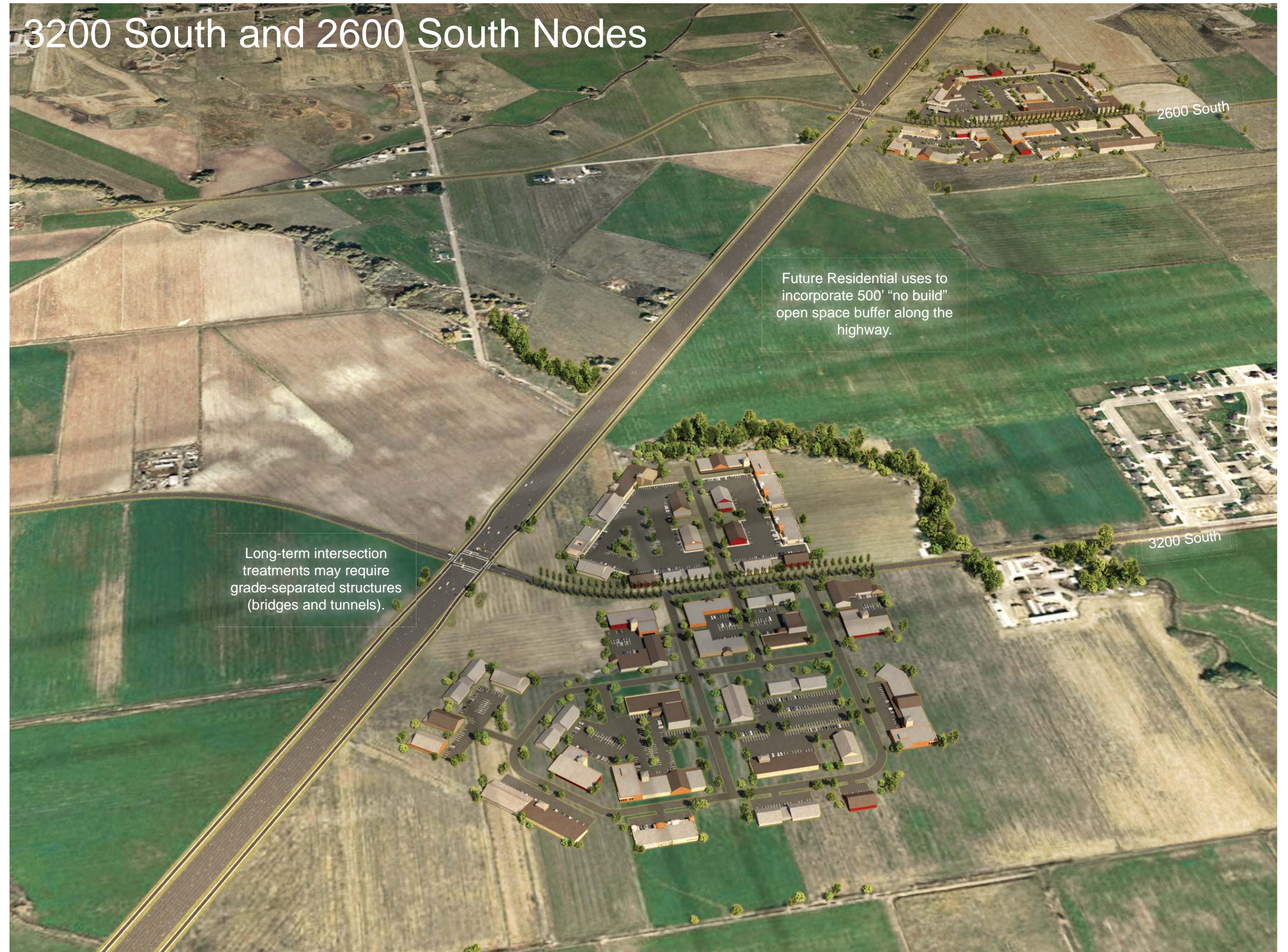
Figure 2-8 Aerial View Above the Nibley Nodes. (Note the consistent 300' setback at the nodes.)
